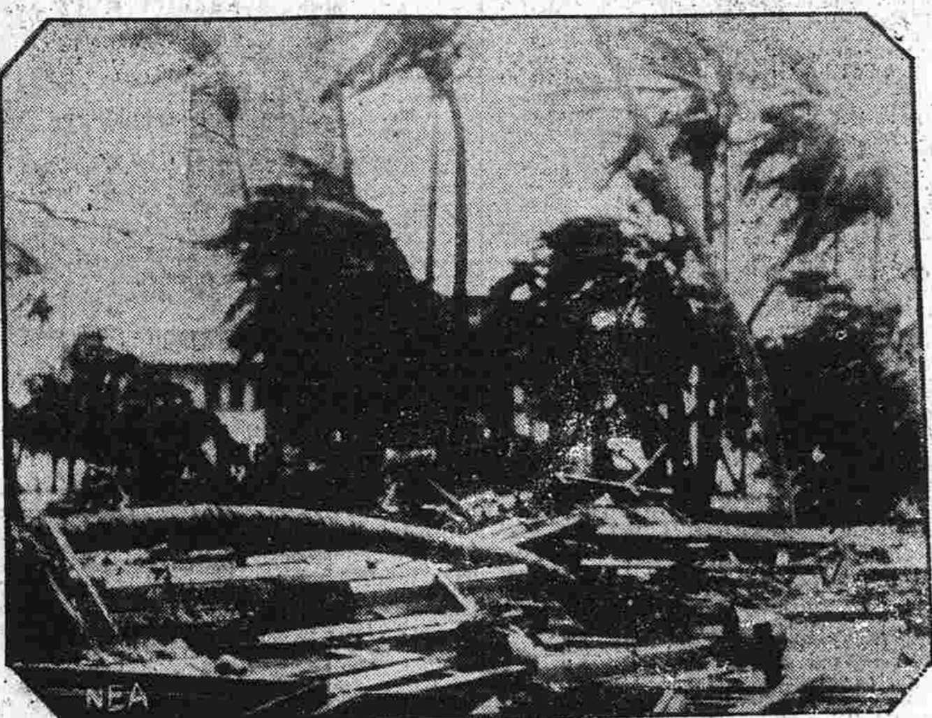
Perhaps better than any other photo does this one show the terrific force of the hurricane as it struck Florida. This NEA picture was taken in the city park at West Palm Beach during the height of the storm. Buildings already had been torn into scattered, twisted wreckage; most of the palm trees had been leveled and the blast. The photographer almost certainly would have been among the casualties had he been in this spot a few minutes before.
